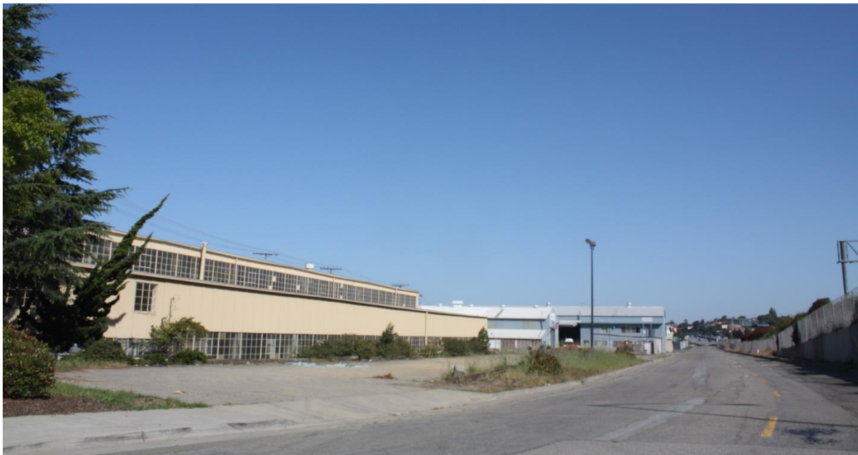
Former industrial building, now in use for tire sales on Cleveland Avenue
