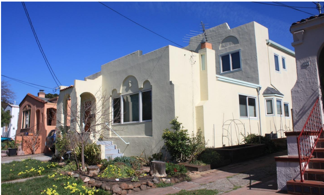
This second story addition incorporates many of the design features of the original home.
