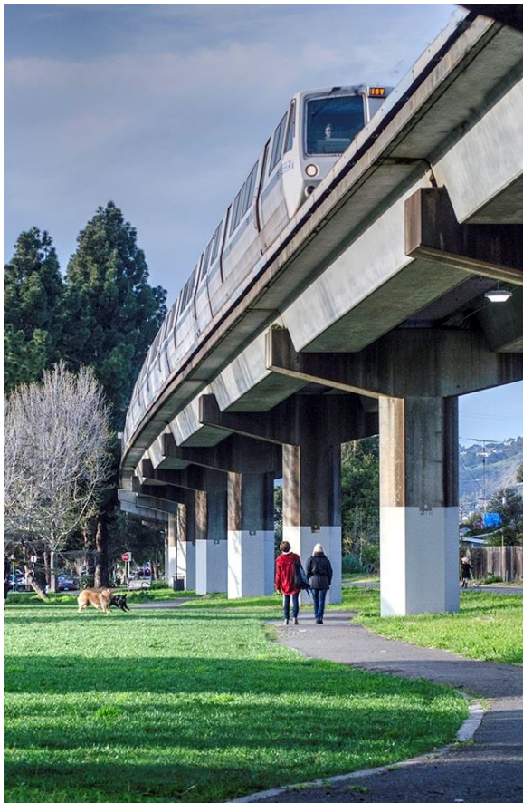
Ohlone Greenway bike trail, with BART tracks above
