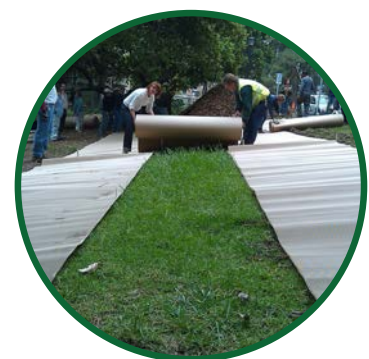
1. Site Preparation & Cardboard Sheet Installation
