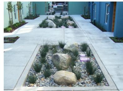
Flow-through planters collect and filter roof runoff in Emeryville.
