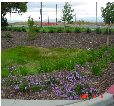
A bioretention area in Fremont detains and infiltrates stormwater runoff.
