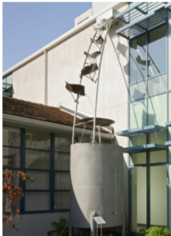
Rainwater is captured and used to flush toilets in Oakland.
