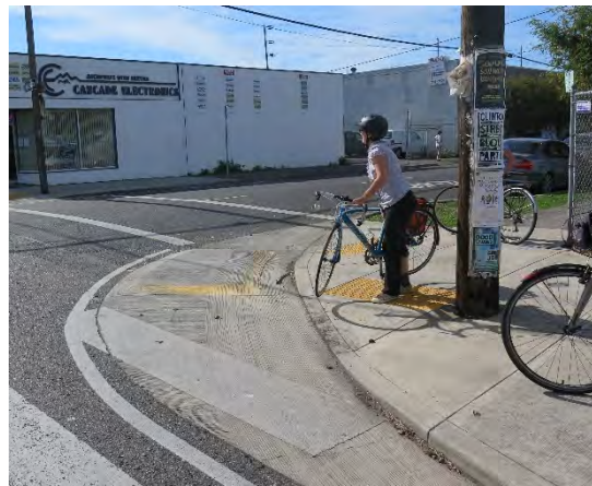
Figure 4.1. Example of the lifecycle of a curb extension: Short-term - temporary installation with paint. Medium-term - concrete repaving without moving the curb line. Long-term - permanent curb extension with shifted curb line.
