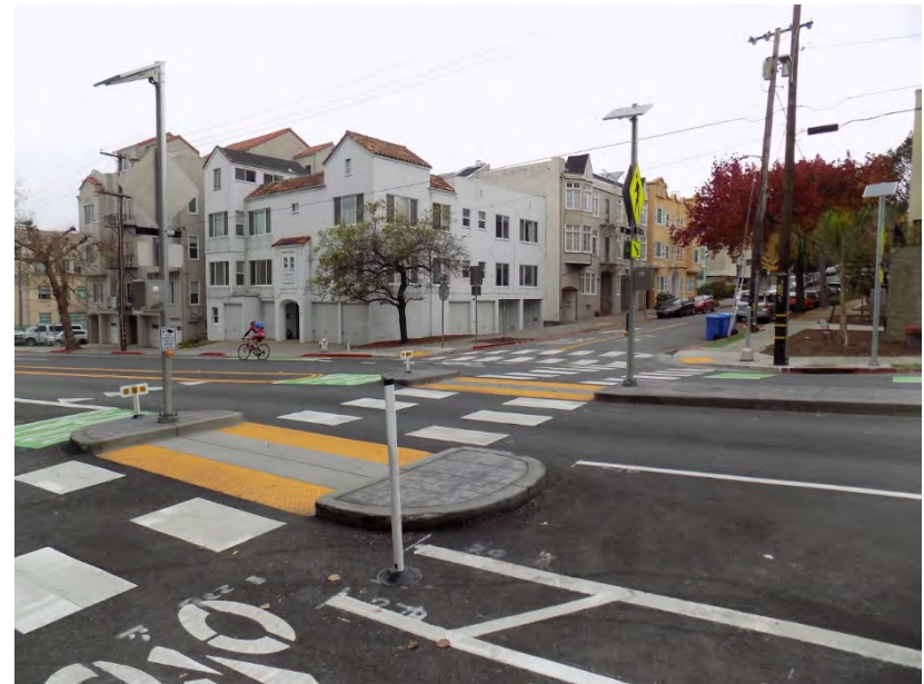
Figure 2.6. A Rectangular Rapid Flashing Beacon at an uncontrolled crosswalk in Berkeley that serves bicyclists and pedestrians.
