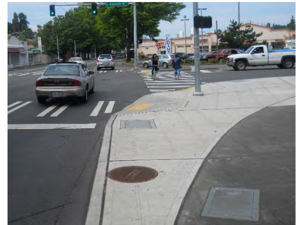
Figure 4.1. Example of the lifecycle of a curb extension: Short-term - temporary installation with paint. Medium-term - concrete repaving without moving the curb line. Long-term - permanent curb extension with shifted curb line.
