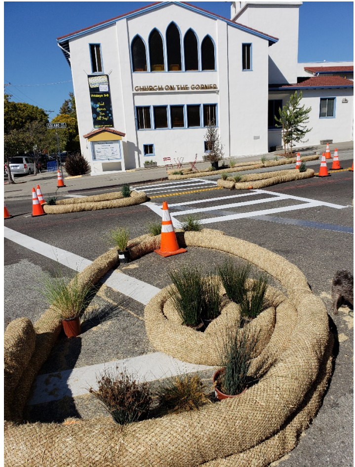
Figure A.5. Temporary materials were used to demonstrate the proposed changes in the proposed corridor design.
