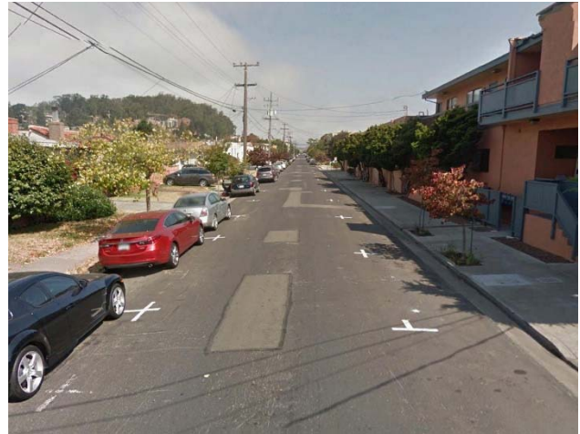
Figure 9 Painted Parking Ts Example
