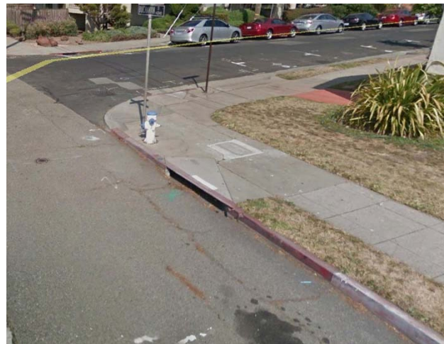
Figure 2 Corner Red Curb
