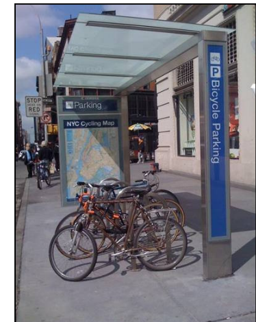
Image I-7: Covered bicycle facility
