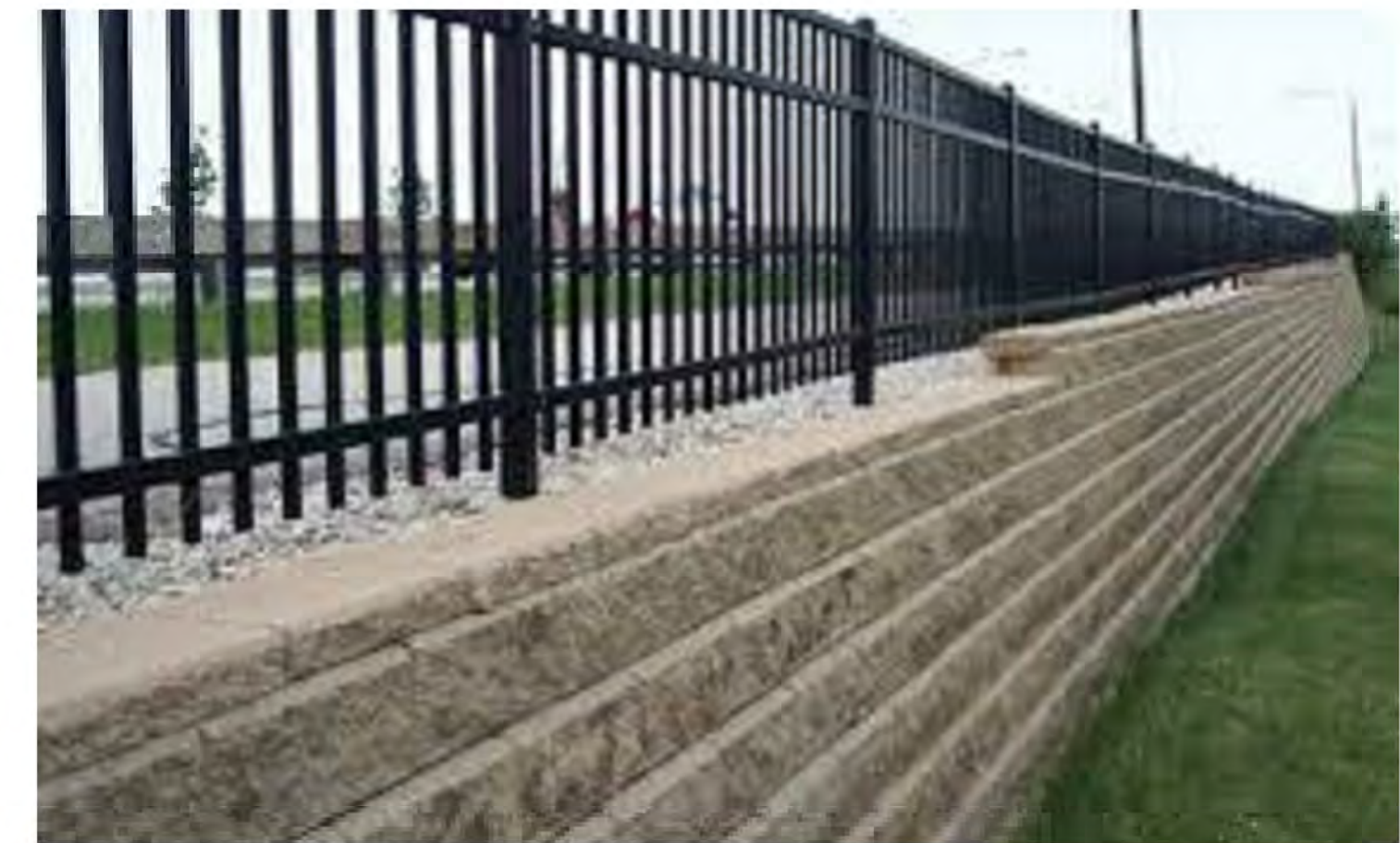
D GRAVITY WALL AND LOW FENCE
