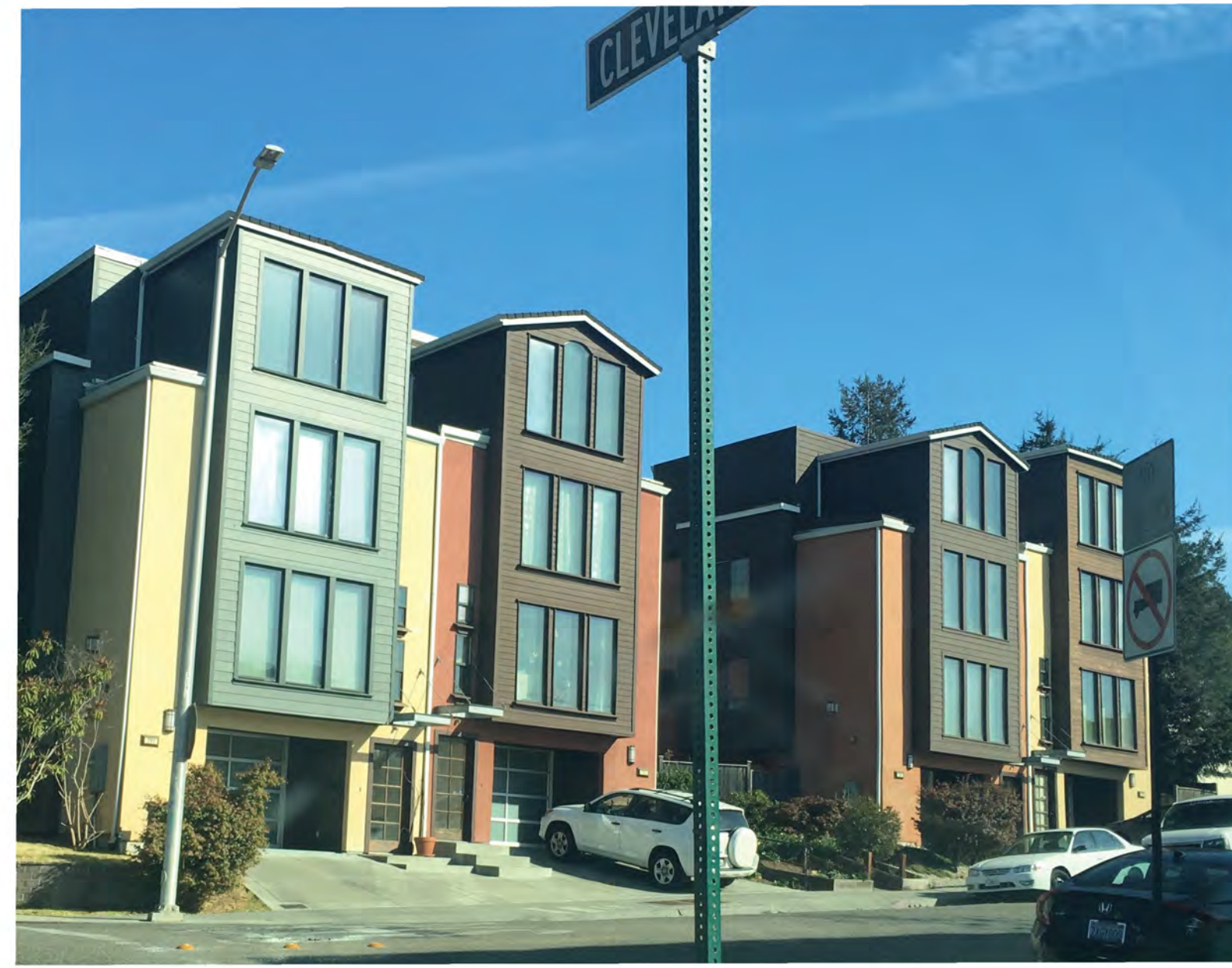
5. VIEW OF SOLANO AVE. TOWN HOMES
