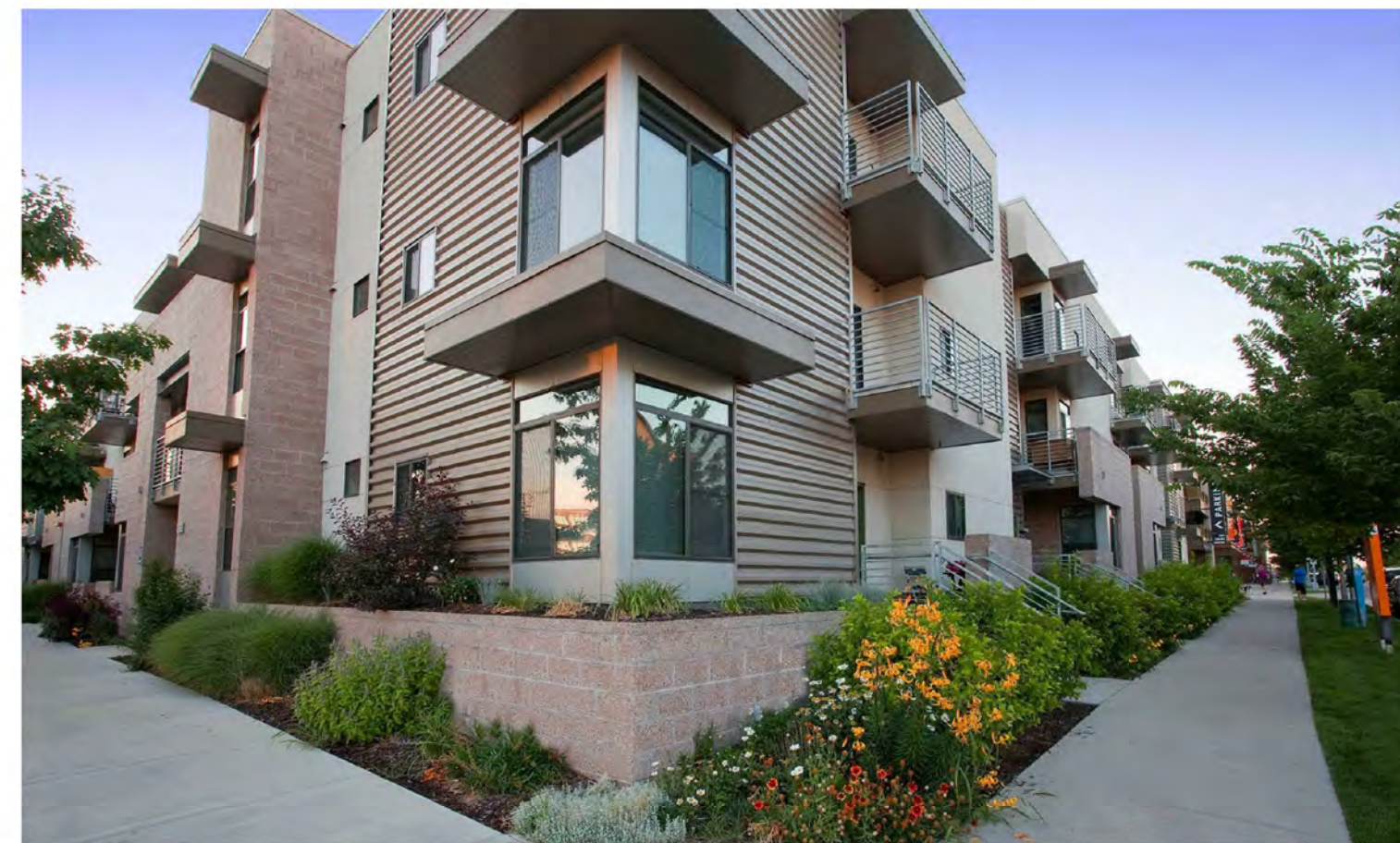
B SIDING & AWNING AT CORNERS
