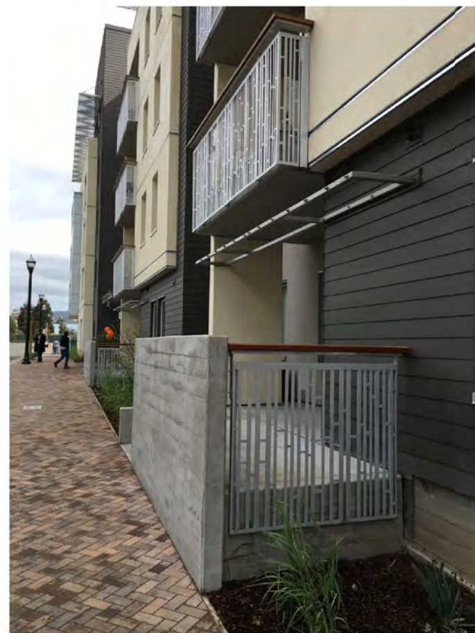
A PERFORATED METAL PANEL
