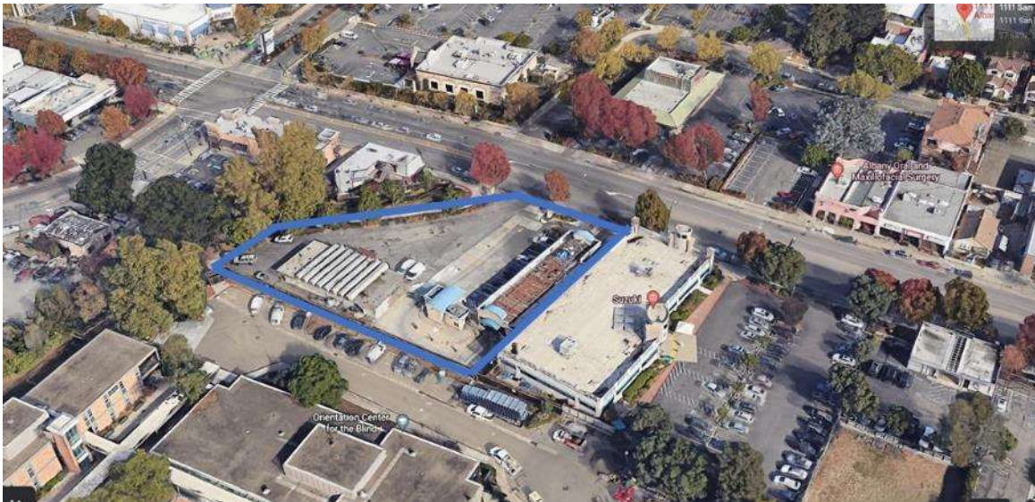
Looking northeast, San Pablo Avenue at top
