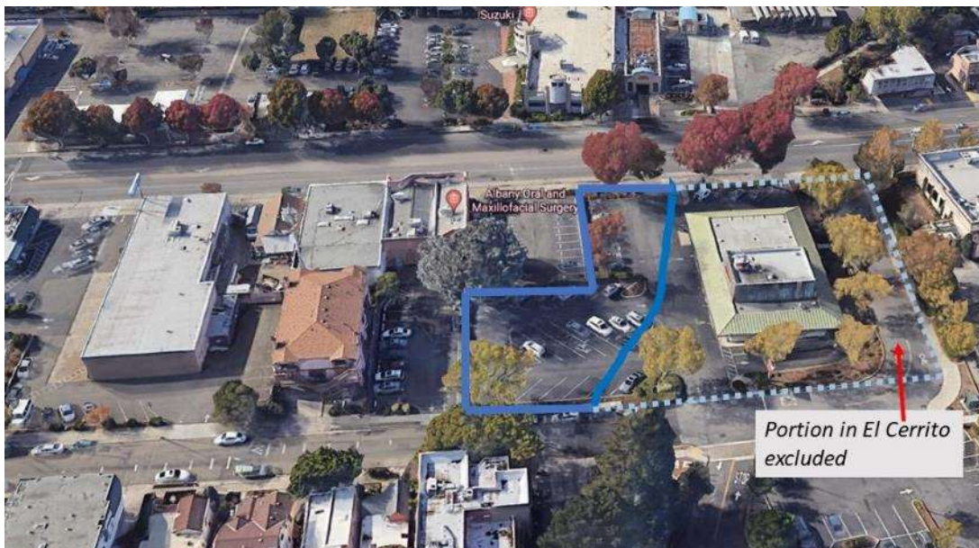
Looking west across Kains Av. El Cerrito portion in dotted blue. San Pablo Av runs across top center.
