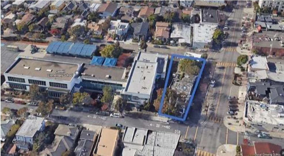
Looking west down Solano across Talbot. Cornell School in center left of photo
