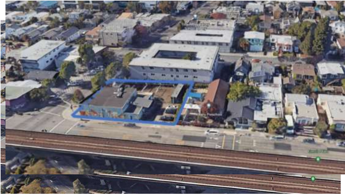
Looking southwest across BART tracks, Solano and Masonic at left
