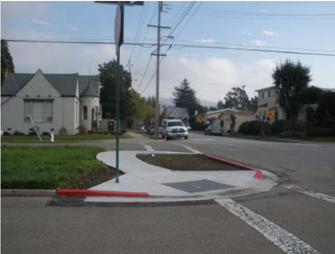
Image 49 – Key Route Median – Crossings
