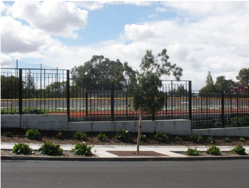
Image 44 – St. Mary's street walls along Posen Avenues
