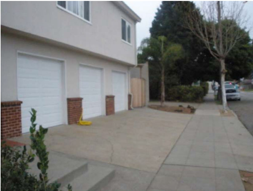
Image 33 –Apartment garages – doors/ façade opportunity here
